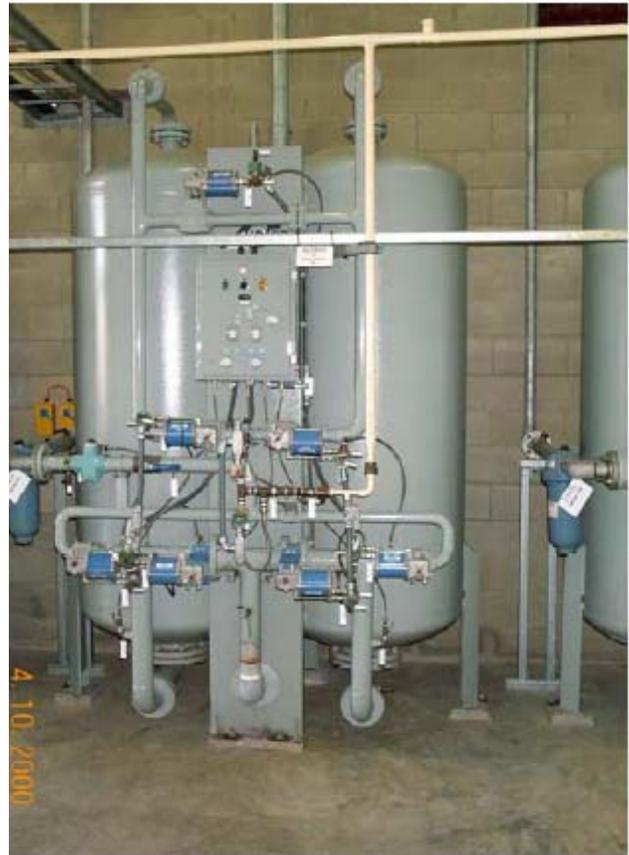
**Figure 7: Detail photos of the ozone generation cells and the PSA oxygen concentrators**
