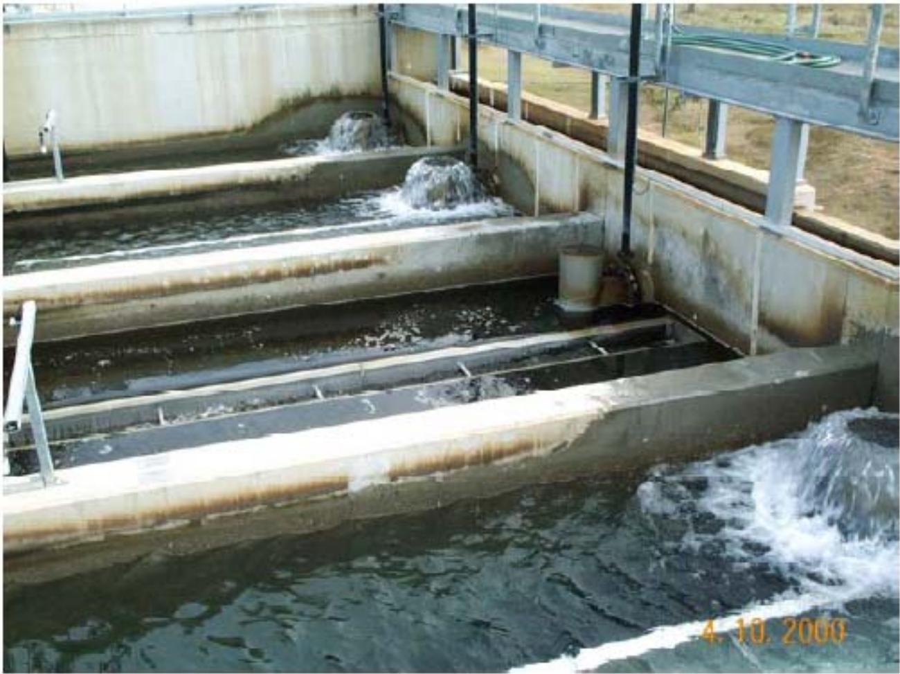
**Figure 8: BAC Unit Process**
