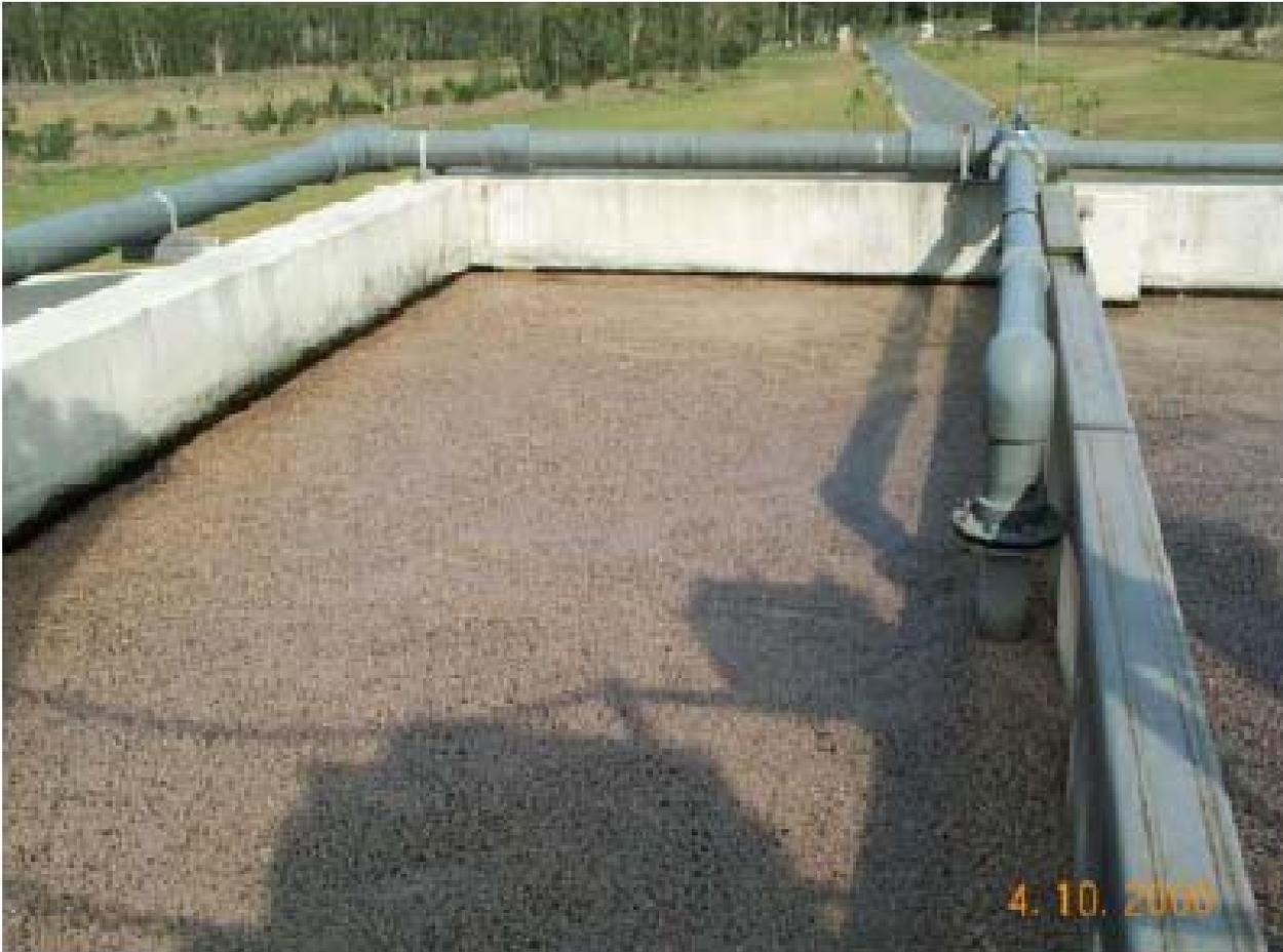
**Figure 5: Denitrification Process Unit**
